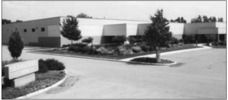
Honeywell's facility in Columbus, Ohio
